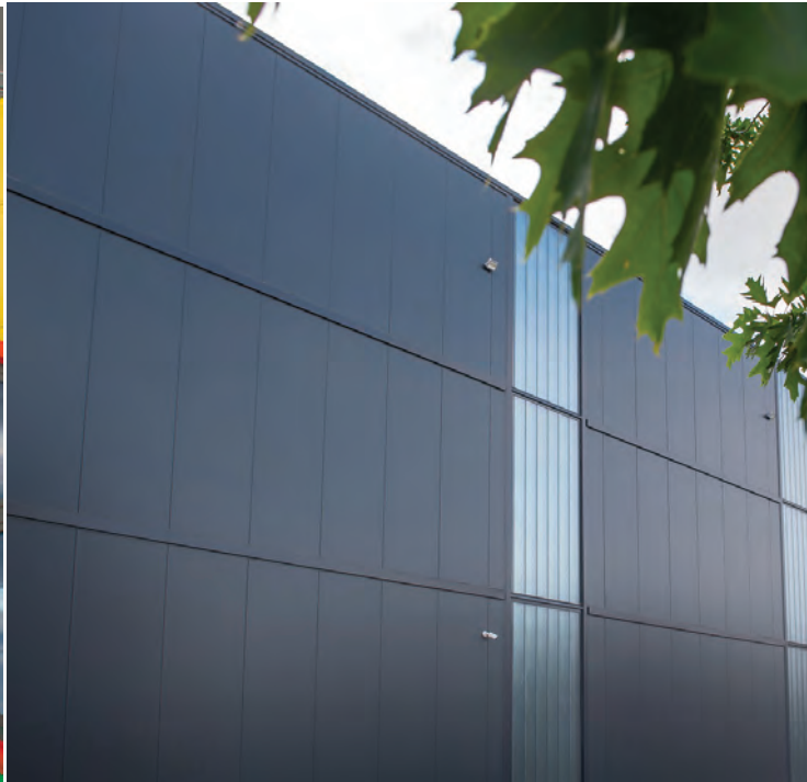
Fot. arch. Adamietz Sp. z o.o.
