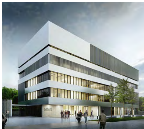
Fot. arch. ROHDE
